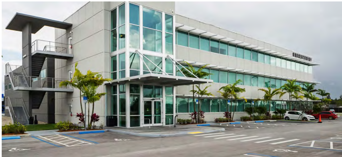
Liebherr offices in Miami, Florida, USA
