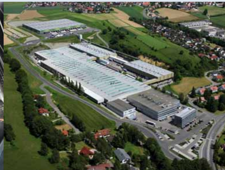
Liebherr Appliances facility in Ochsenhausen, Germany
