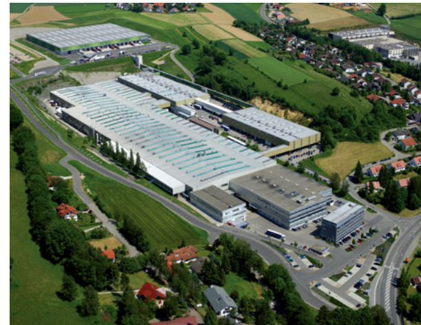
Liebherr Appliances facility in Ochsenhausen , Germany
